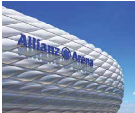
Allianz Arena - Munich, Germany Engineer: formTL Fabricator: Covertex Labor Blum: German approval (Z.i.E.), production inspection
