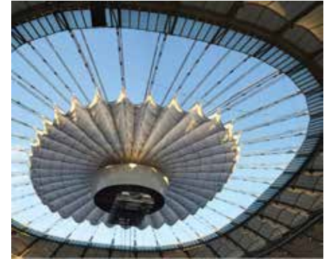
BC Place - Vancouver, Canada Engineer: sbp GmbH Fabricator: Hightex GmbH Labor Blum: Quality control for the inner roof
