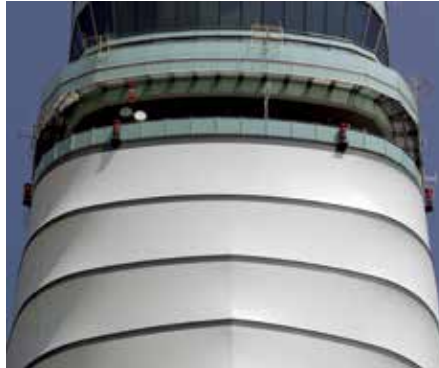
Airport Tower - Vienna, Austria Engineer: Peter Mandl ZT GmbH Fabricator: Covertex Labor Blum: Material expertise
