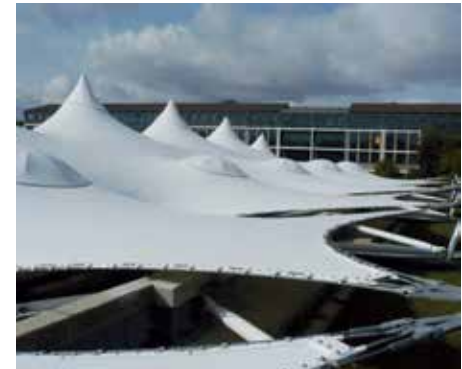
Forum Montrouge - Paris, France Engineer: IFgroup Fabricator: Graboplan Labor Blum: French approval (Atex), quality control, biaxial testings, membrane stress measuring
